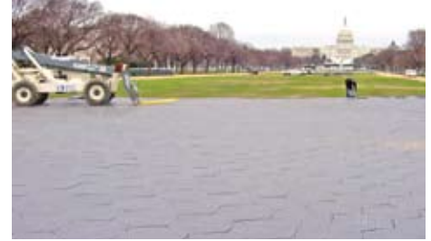
HexaDeck in use on the National Mall for the 2005 Presidential Inauguration.
